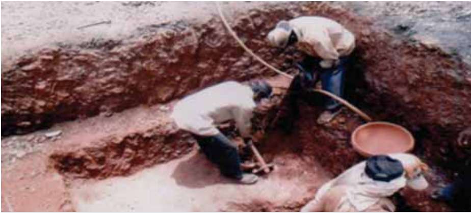
Construction Work in Progress at the Project Site
